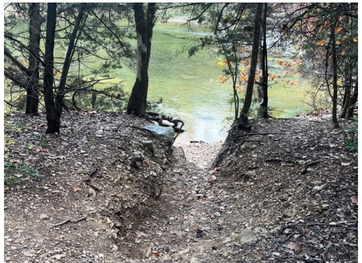
GULLY EROSION near Hill of Life Dam.
