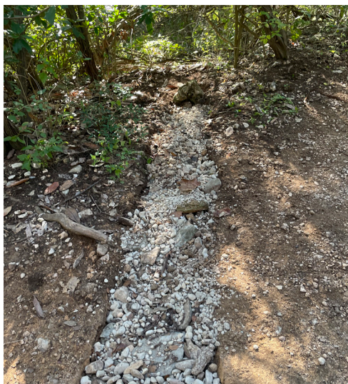
Grade dips back filled with gravel installed to mitigate sheet and rill erosion frequently occurring in low areas on trail. ▶
