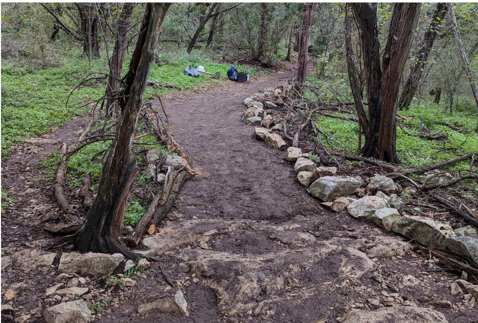
Rocks and brush used to delineate a more narrow path in a wide segment of trail. Edges were seeded with inland sea oats ▼
