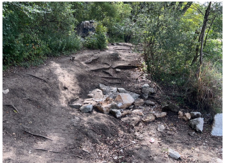
BANK EROSION near Gaines Creek Trailhead.
